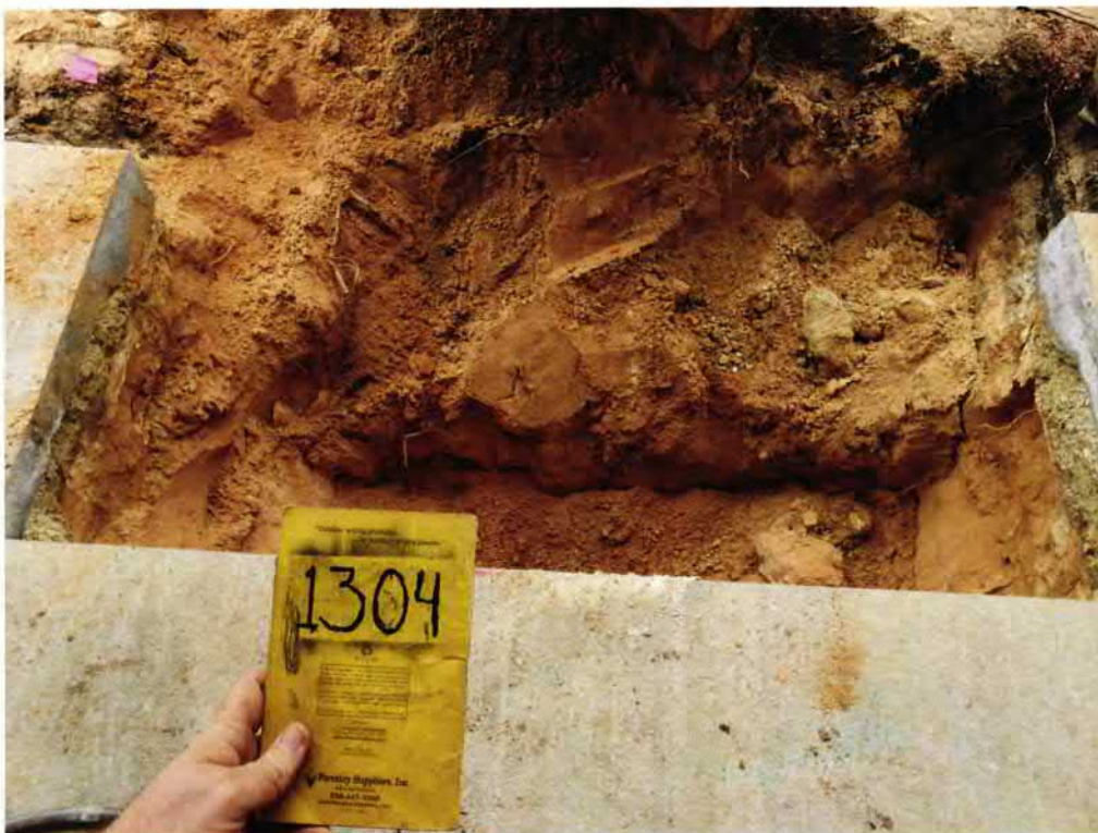
Picture 2: UST 1304Eagle excavation.
